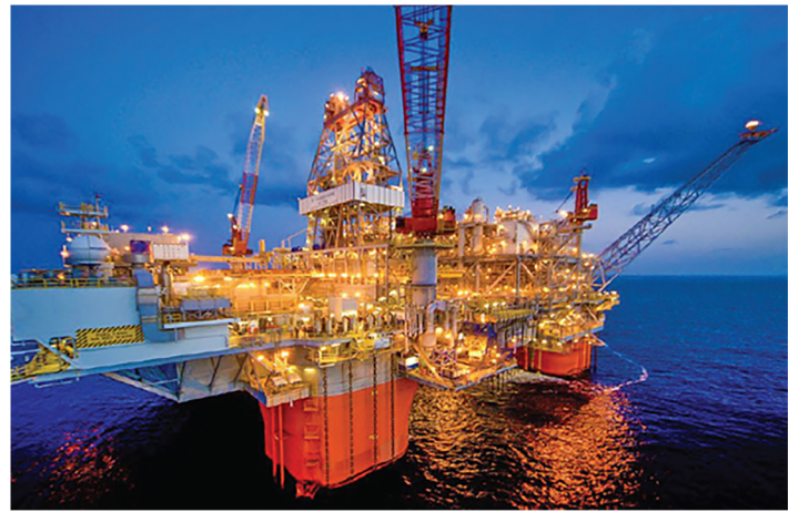
12 Ocean Oilfield Drilling Rigs Location: Sharjah-UAE
